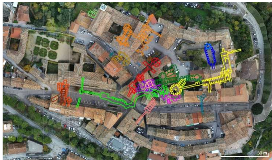
Figure 1. Overview of the city center of Camerano (Italy) with overlaid the map of the underground caves (ca 3 km long).
