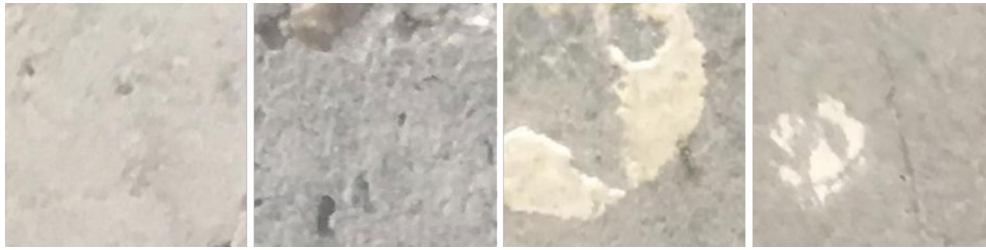
Fig. 5 Negative crack images from Concrete Crack Images for Classification dataset (Özgenel 2019)
