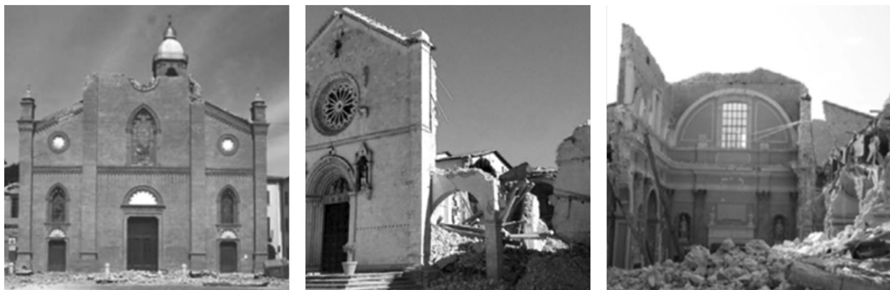
Fig. 1 Example of damage that occurred to churches hit by past earthquakes: a) St. Maria Maggiore Church in Mirandola (Emilian earthquake, 2012); b) St. Maria Paganica Church (L'Aquila earthquake, 2009); c) St. Benedetto di Norcia (Norcia earthquake, 2016/2017)
