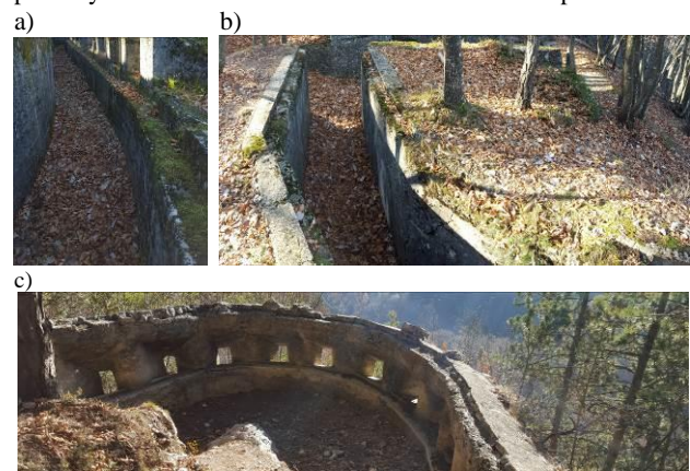
Figure 9. The excavated trench connected to the tunnels and artillery batteries in caves (a, b) and a rifle emplacement (c).
