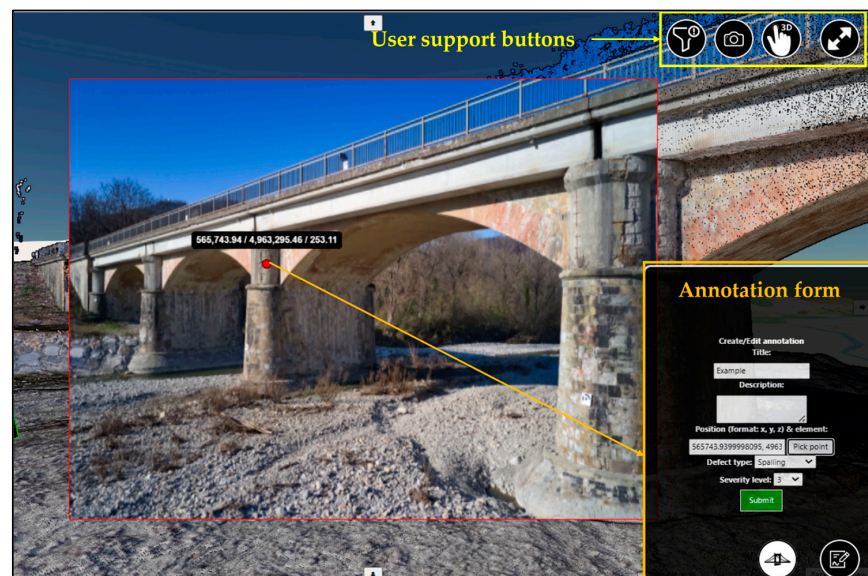
Figure 9. The interface allows users to inspect a textured 3D model of the bridge and record defect annotations by selecting a point directly on the geometry. Each annotation captures spatial coordinates, defect type (e.g., spalling), severity level, and optional textual descriptions. This integration facilitates consistent documentation and streamlined condition assessment in a spatially aware environment.
