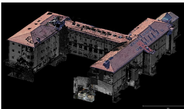
Figure 6. The complete point cloud of the B6 building.
